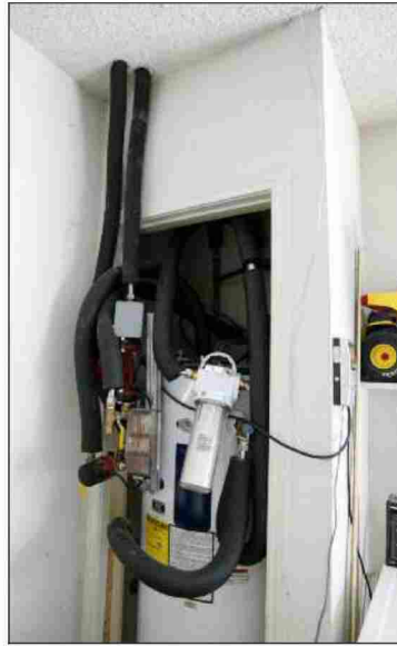
This is what the solar water heating system looks like inside the Below house.
